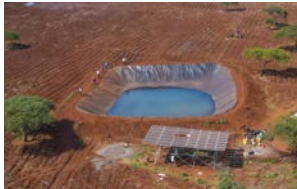
Solar irrigation system
